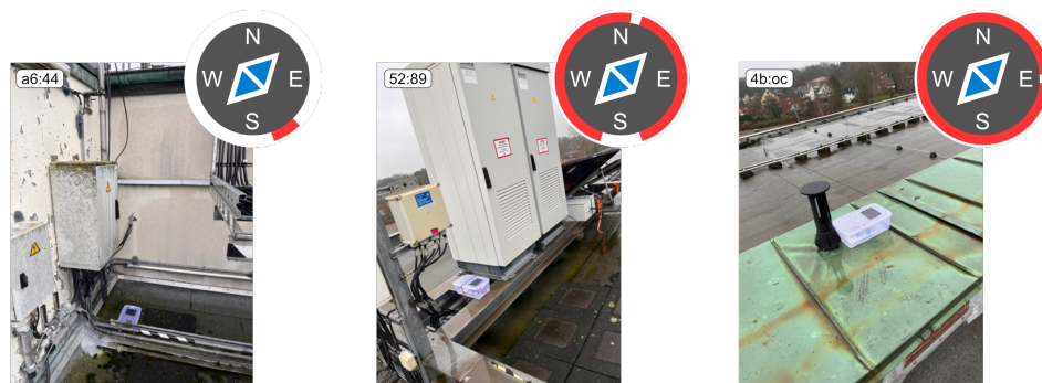
Figure 7.8: Positioning of the prototype solar modules for the second scenario, with respective pseudo-compasses to show the irradiation angles.
